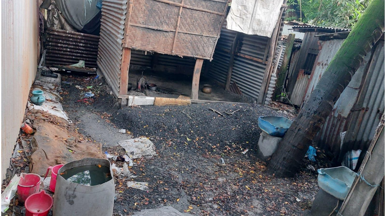
Figure 5: Hazardous Outdoor in front of a Metallic Workshop
